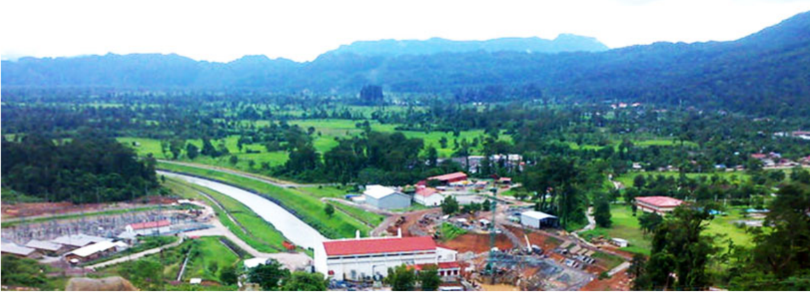
Theun-Hinboun Switchyard 1 image below:
